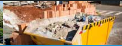
Pre & Post Construction Cleanup
